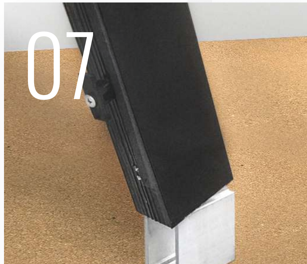
Install vertical profiles as shown in the photo.
