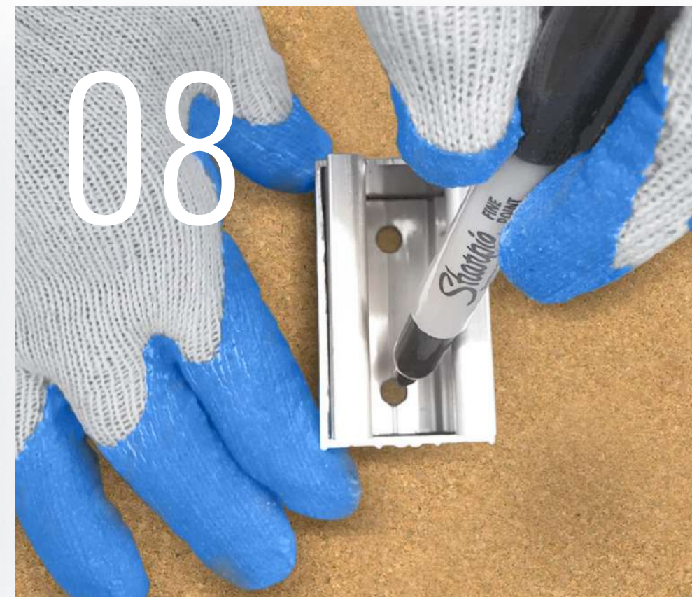
Using F10 Floor Bracket Setup mark screw location.
